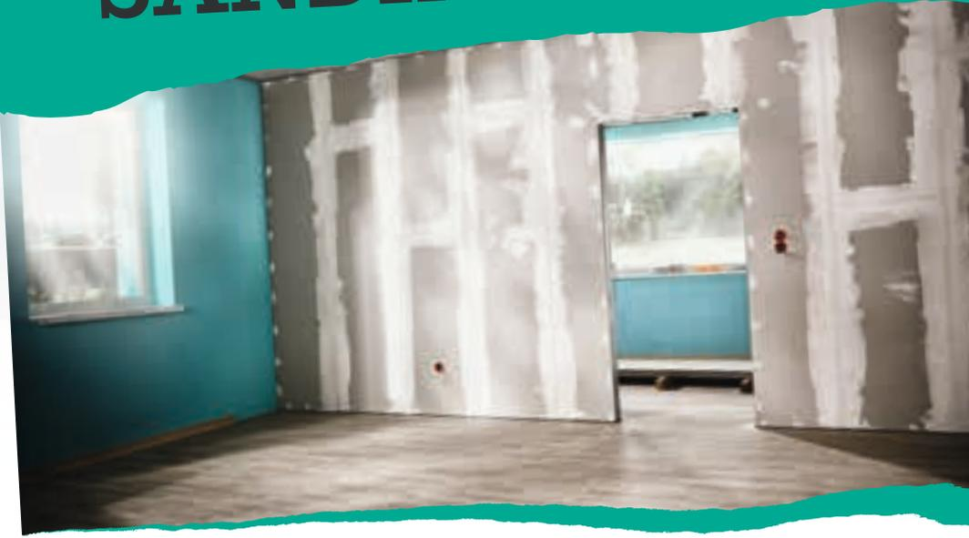
Now most of the hard work is done, you can focus on fine sanding. In order to achieve a smooth surface finish, the joints between the plaster boards in particular require thorough sanding with the hand-held grinder. Here it is important to make sure that the cardboard layer is not damaged. **wolcraft** has developed the ergonomic 225 mm **surface sander** for quicker sanding progress and greater stability when working on walls.
