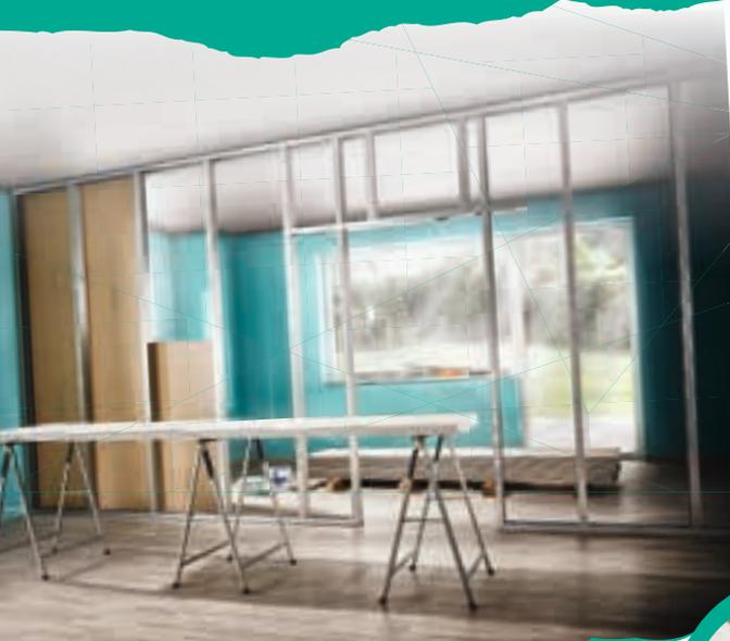
The stud frame has been erected, the plasterboard cut to the correct dimensions and the wall is slowly taking shape. You should provide a gap below the plasterboard adjacent to the floor. Universal wedges from *wolcraft* are a worthwhile investment that will pay dividends in countless situations such as this.
