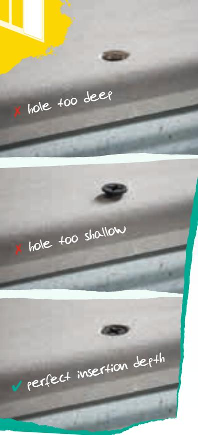
The screw heads should be countersunk slightly so that they can be plastered over easily at a later stage. Caution: Do not drill too deep, otherwise you will damage the cardboard layer and the screw will no longer grip properly. If you want to be absolutely sure:
