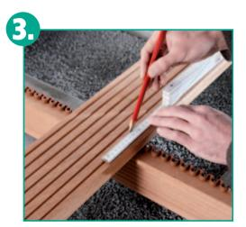
Mark both drilling and screwing positions with two lines on the upper side of the deck board and take care that the borehole is not positioned in a groove of the board.
