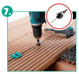
Having spot-drilled the boreholes, put the drilling guide aside and finish drilling the boreholes. The countersinks for the screw heads are done in the same way. The depth of the countersink can be set precisely with the screw starter with countersink and depth stop.
