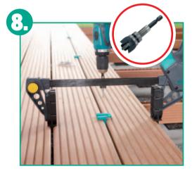
Once all boreholes have been drilled into the deck board, screw the board with the magnetic bit holder to the centre of the supporting girders. Slightly bent deck boards can be straightened with the installation clamp without any problems.
