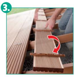
Hint: You may have to pre-drill boreholes in hard wood so as to prevent the wood from cracking or the screws from breaking off. Please make sure that the floor board cannot slide away while being screwed to the joiners. The joiners will now protrude from both edges of the board. Once all joiners have been fastened, the board can be turned upside down again.
