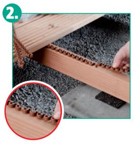
If necessary, the **distance bars** can be extended by positioning them together at their ends or they can be shortened as required. The deck boards themselves will later be screwed to the centre of the joist, so as to prevent the joist from tilting.
