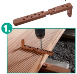
Just put the last floor board (upside down again!) flush onto the previous floor board and mark the outer edge of the previous joiner with an angle on the last floor board. Align the joiner with this line and fix it with four screws.
