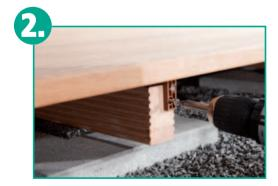
Then turn the board over again and push the joiners under the previous floor board, as before. And finally, fasten the joiner with two screws to the front edge of the joist.
