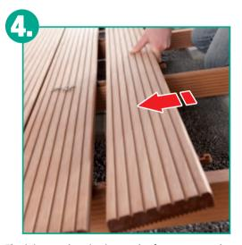
The joiner end projecting to the front can now be pushed under the previous floor board which will arrest the board automatically at its front edge, while it will still have to be fixed at its rear edge with two screws. The joiners will also act as spacers between floor board and supporting joist and prevent water logging, which otherwise would unnecessarily accelerate the rotting of the wood.
