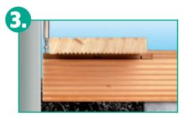
You can now put the board with the shortened joiners flush to the wall of the house, thus leaving a gap of 1 cm between the wall and the edge of the board. This is enough space to fix the floor board to the joist using one screw for the rear borehole and two screws in the front section.
