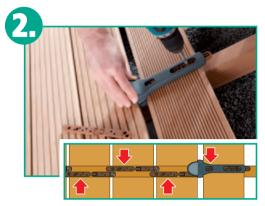
Put the back of the floor board upside down against the previous board and align it flush towards the front end. Place the drill gauge onto it and align it rectangularly to the floor board. The drill gauge can be placed immediately next to the previous joiner with the help of the two stops (arrows in Fig. 1), either on the left or on the right-hand side
