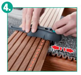
Put the **drilling guide** onto the deck board and adjust the rear drilling bush with the help of the notch on the side, so that it hits exactly the relevant marking line.
