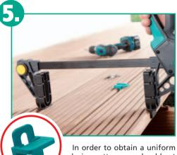
In order to obtain a uniform laying pattern, you should put a **spacer** between the floor boards every 80 - 100 cm, choosing a distance of either 6 or 8 mm bet-
