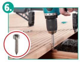
... and fixed safely with the first-class stainless steel screws supplied. The special installation clamp comes with two additional clamping jaws, so that it can be used as practical one-hand clamp at any time.
